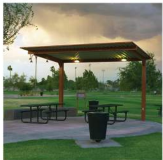
OVERHEAD SHADE STRUCTURE
