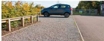
PERMEABLE PARKING LOT
