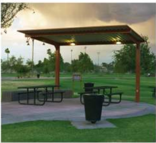
OVERHEAD SHADE STRUCTURE
