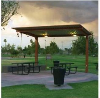
OVERHEAD SHADE STRUCTURE
