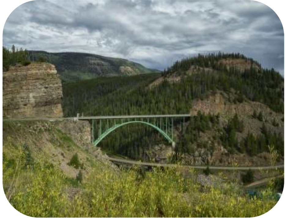
Red Cliff Bridge, Eagle County
