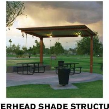
OVERHEAD SHADE STRUCTURE
