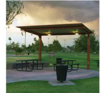
OVERHEAD SHADE STRUCTURE
