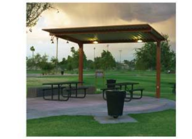
OVERHEAD SHADE STRUCTURE
