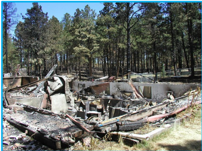
The unburned trees in the background show that this home, burned in the Black Forest Fire, was not engulfed by flames. Rather windborne firebrands ignited the home.
