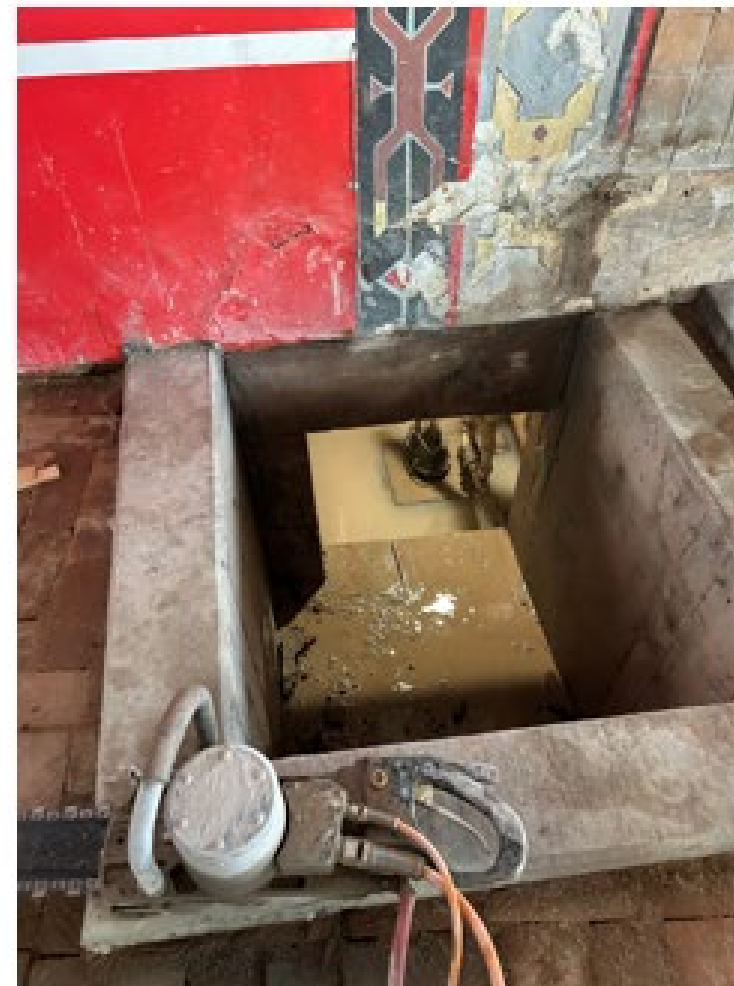
Addition of exterior access
