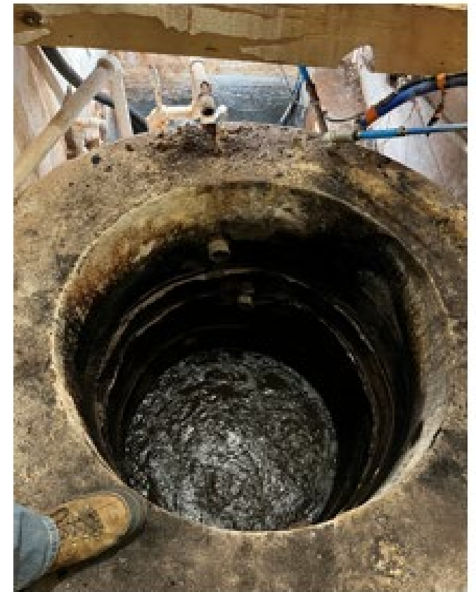
Gas bell removed
