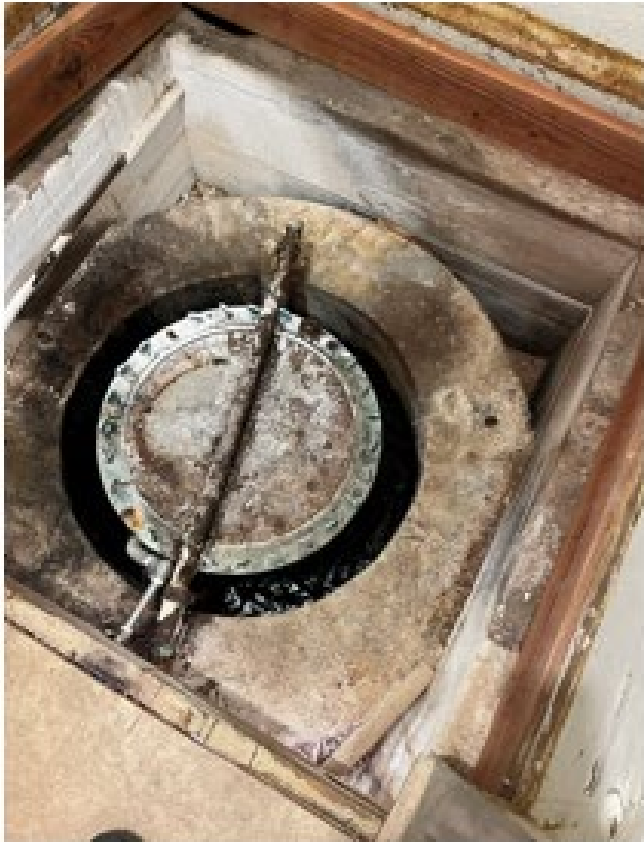
Gas bell in place
