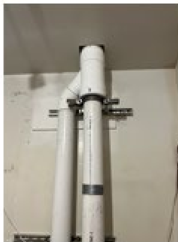
Venting and Framing
