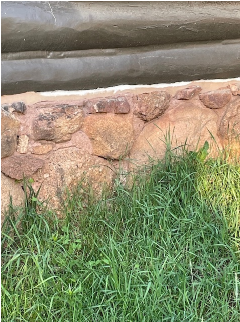
Natural stone foundation
