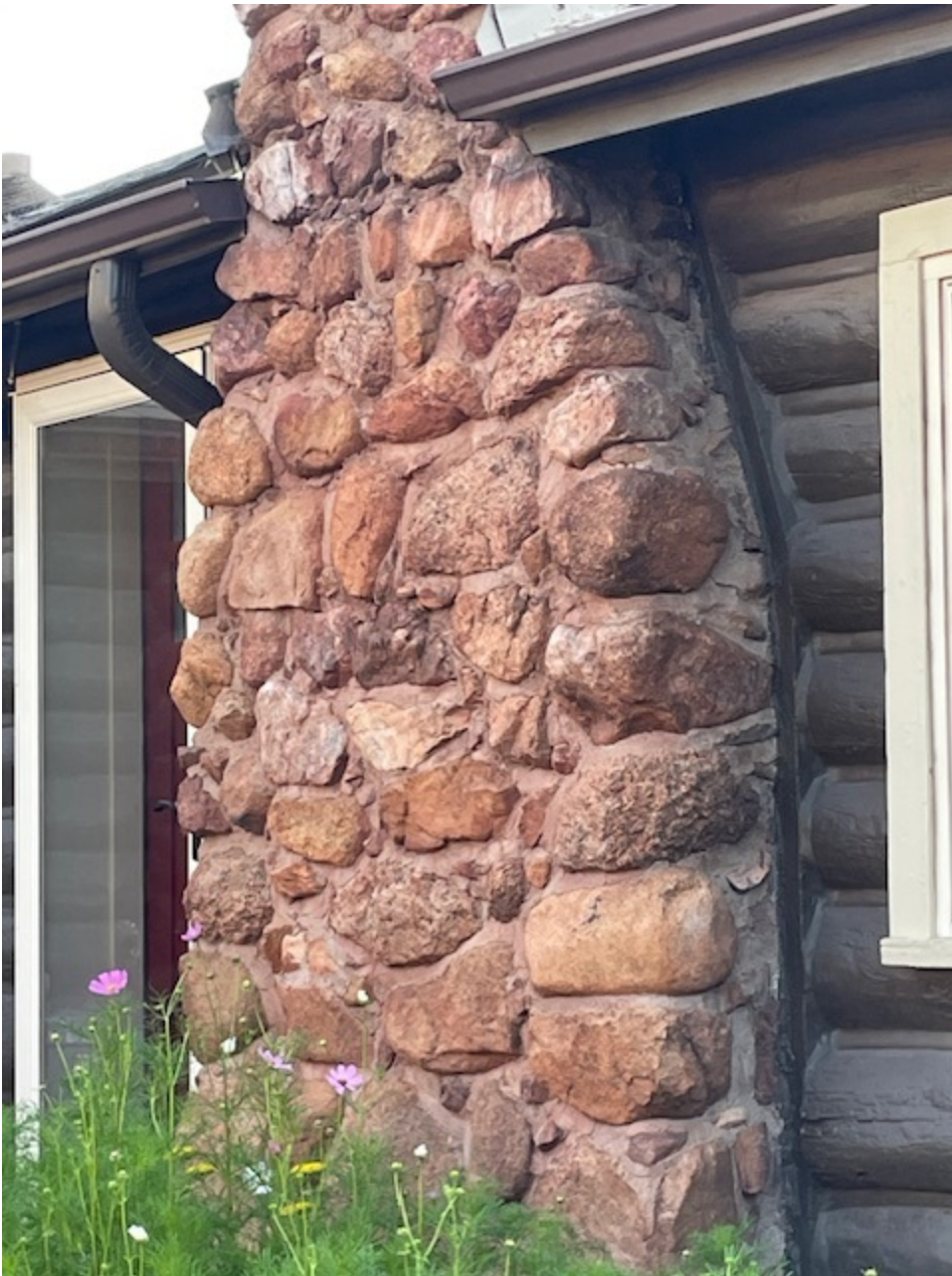
Natural stone chimney
