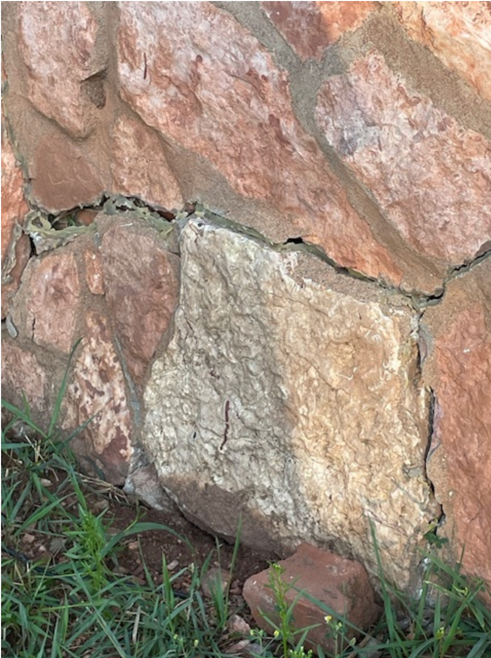
Failing mortar
