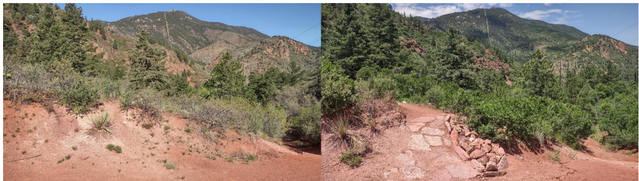
Figure 2: Before (left) and after (right) of rock armored ramp at the reroute entrance.
