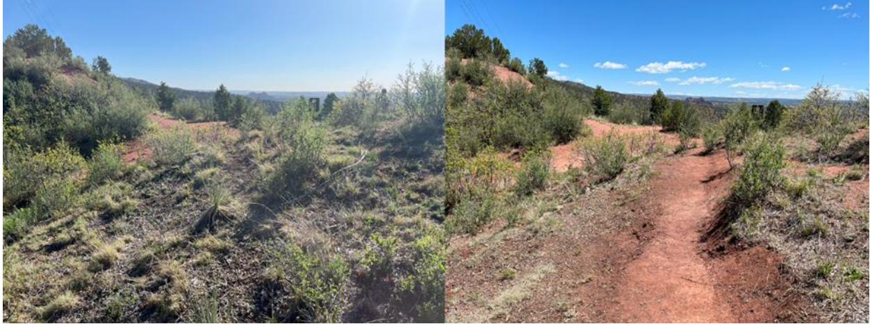
Figure 3: Before (left) and after (right) of Intemann Trail reroute.
