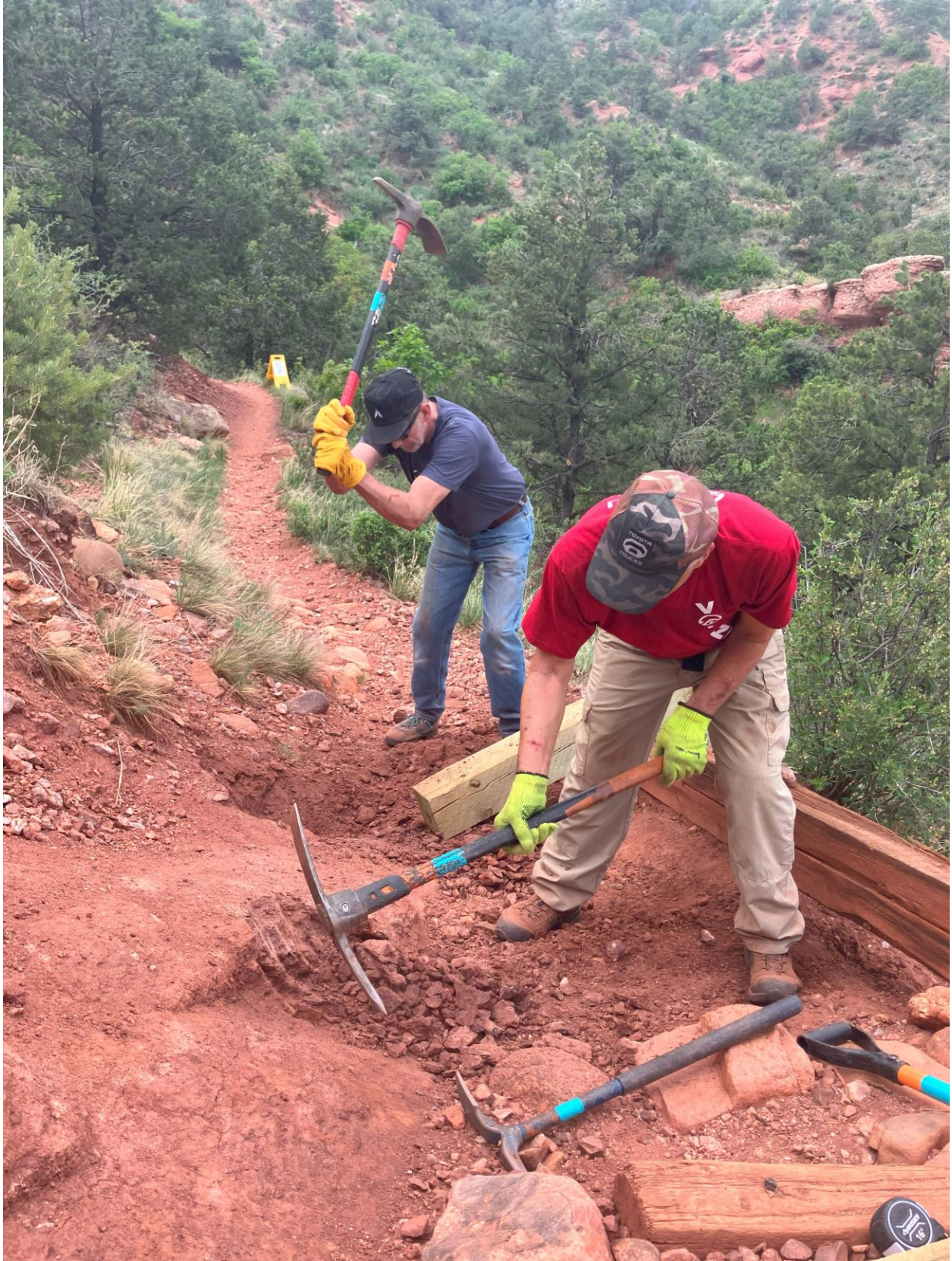
Figure 10: Volunteers repairing the failing timber structure.
