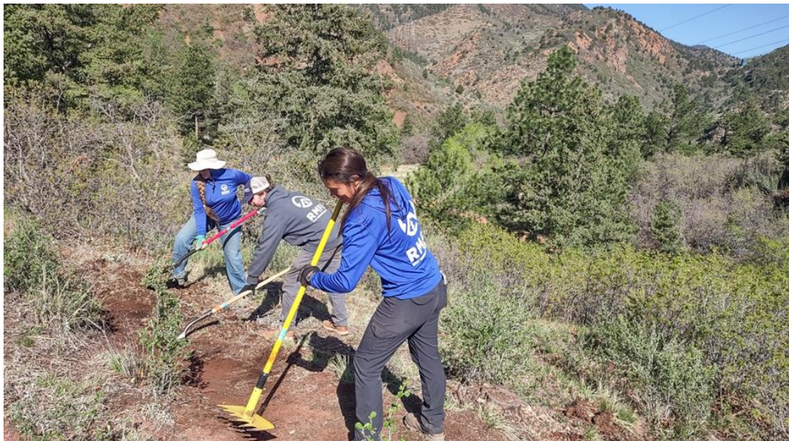
Figure 7: RMFI crew digging and refining the new trail.
