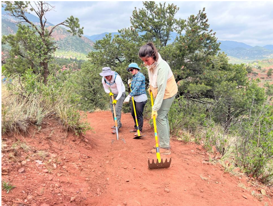
Figure 9: Volunteers removing the berm and building drains.
