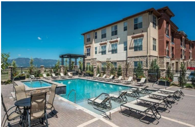
Vue 21 Apartments – Colorado Springs
