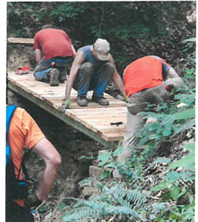
Building a bridge 1 mile deep into Yellowwood State Forest
