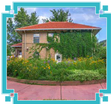
Manitou Springs Carnegie Library
