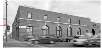
McPhee and McGinnity Building Addition
