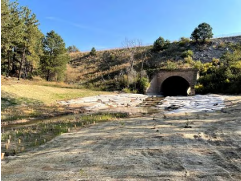
Figure 1 Example Sculpted Concrete Structure
