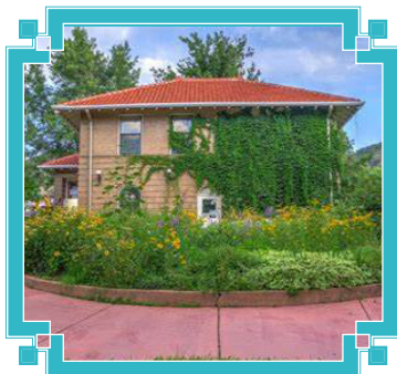
Manitou Springs Carnegie Library
