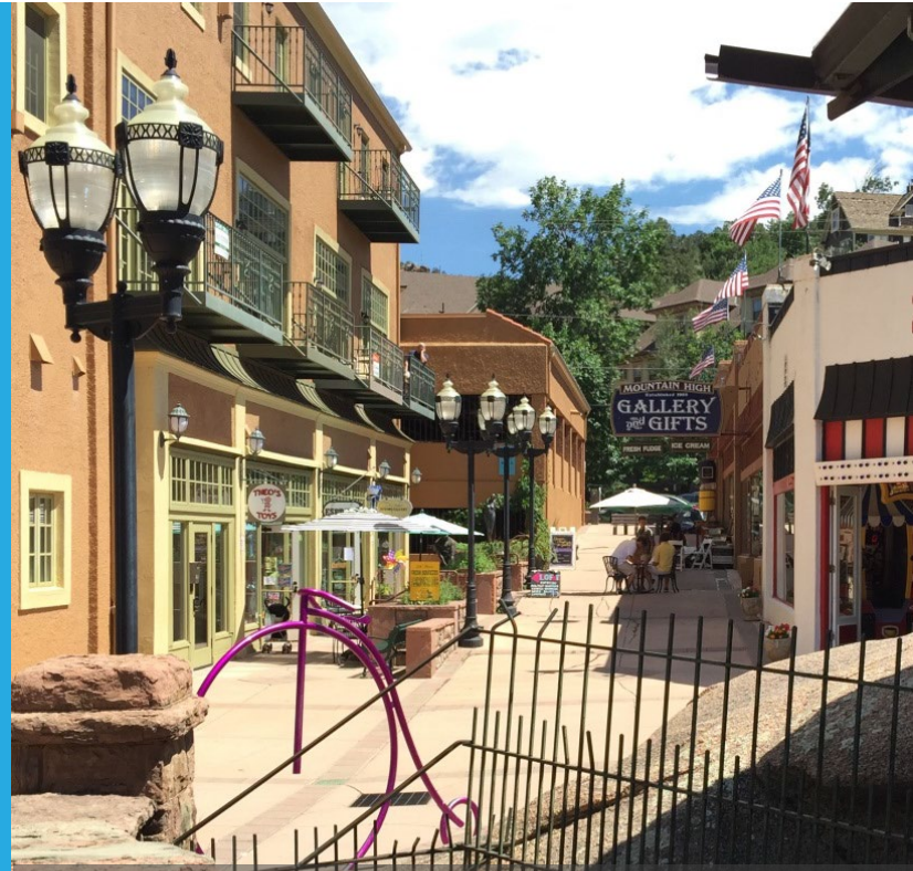
The Spa Building in Downtown Manitou Springs is a renovated historic structure that contains a mix of uses – Photo courtesy of Clint Hager
