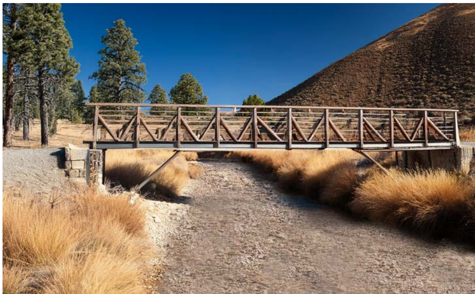
PEDESTRIAN BRIDGE TO TRAILHEAD
