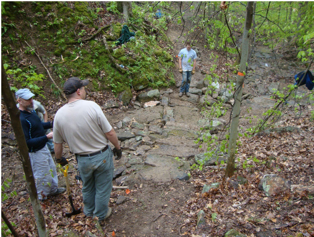
Armoring Project with Park Staff, Americrops, and local volunteers
