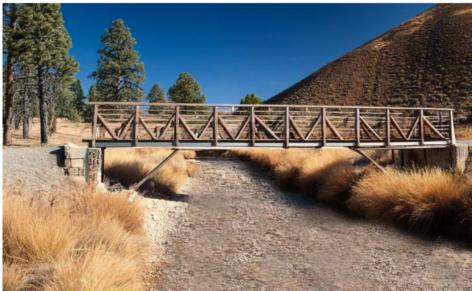
PEDESTRIAN BRIDGE TO TRAILHEAD
