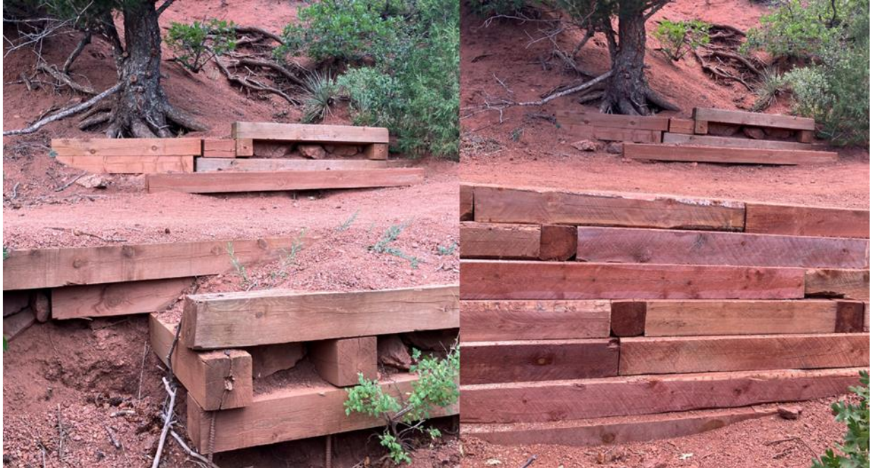
Figure 4. Before (left) shows the old failing timber structure. After (right) shows the new timber retaining wall.
