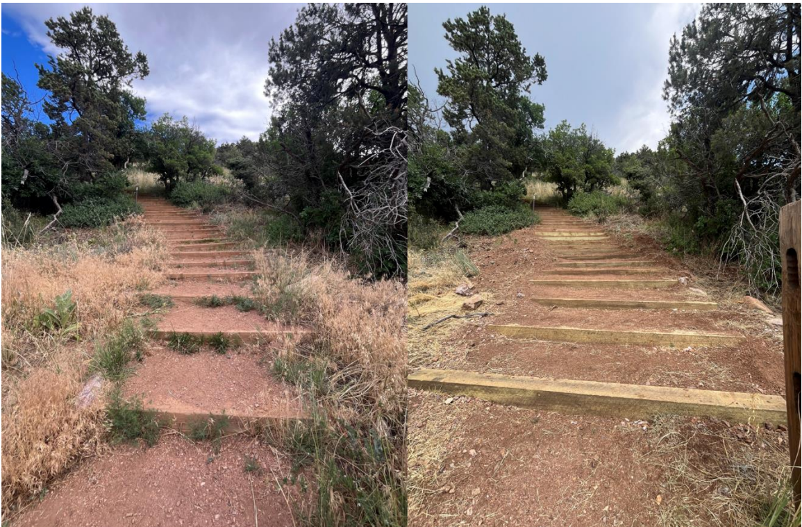
Figure 8. Before (left) and after (right) of the upper single riser timber steps that were replaced.
