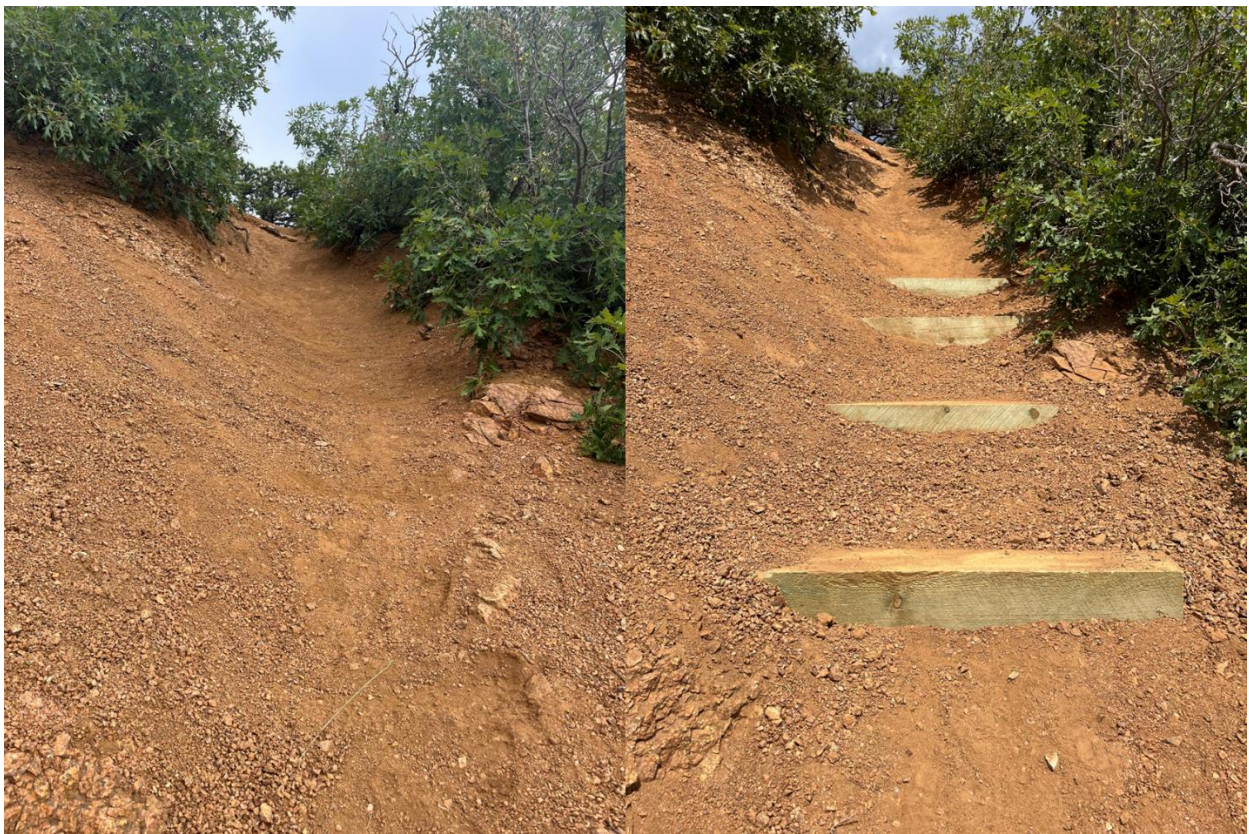
Figure 2. Before (left) and after (right) of timber steps at Red Mountain trail.
