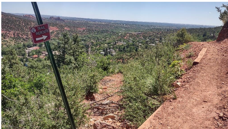
Figure 6. Restoration worksite for future work.
