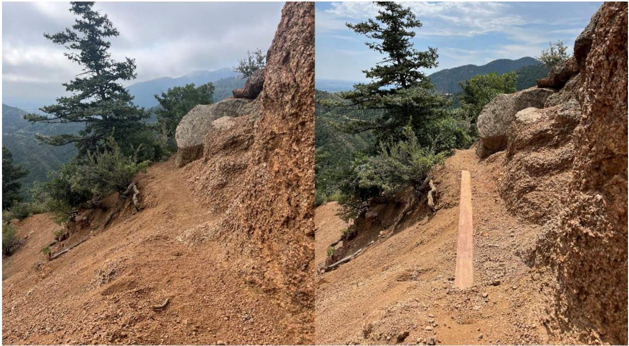
Figure 1. Before (left) and after (right) of single log retainer at Red Mountain trail.
