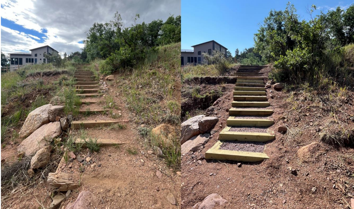
Figure 7. Before (left) and after (right) of the southern set of timber steps that were rebuilt.
