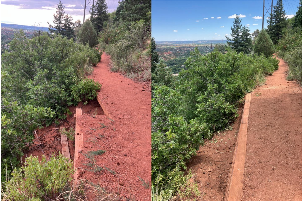
Figure 5. Before (left) and after (right) of timber retaining wall and tread work.
