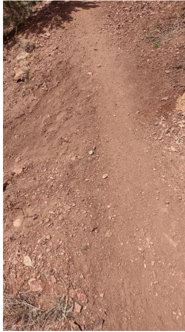
Figure 9. Critical edge of trail eroding in this area.
