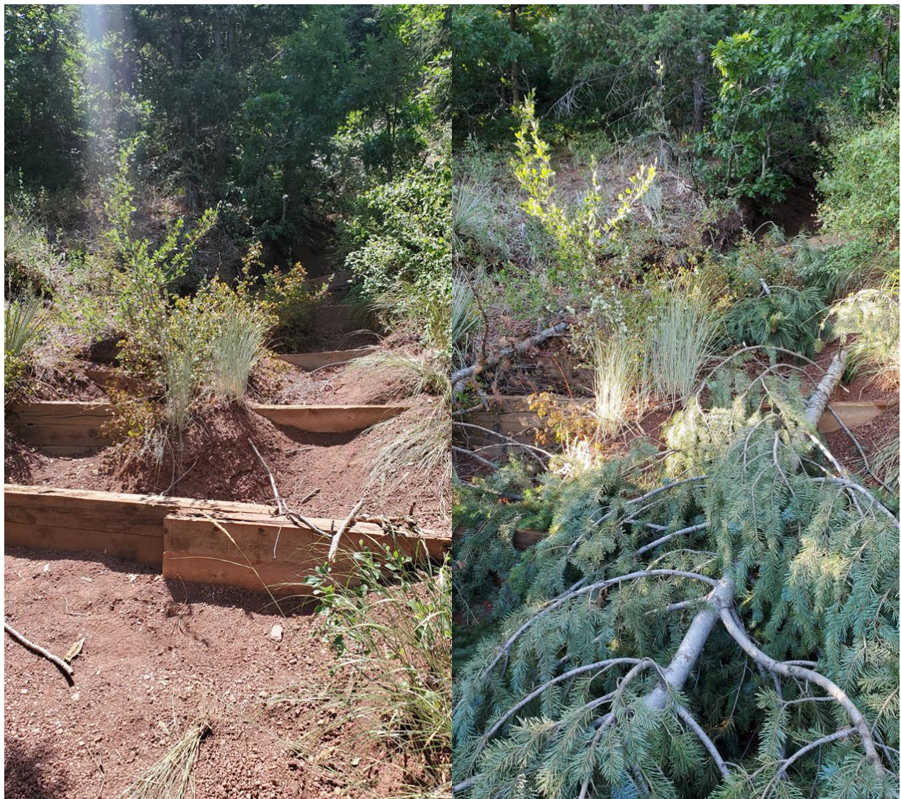
Figure 3. Left shows the gully after timber check dams were installed. Right shows the site covered with slash and disguised.
